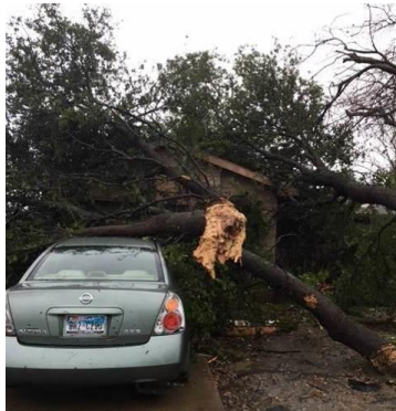
Tornado damage in Rowlett, Texas.
