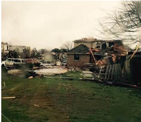
Tornado damage in Rowlett, Texas. Photo: Liz Disco-Shearer
